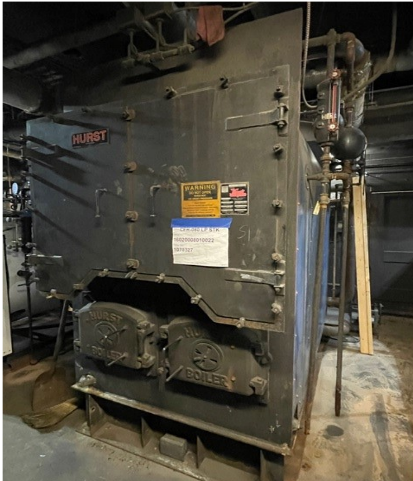
Out with the old coal fired boiler
