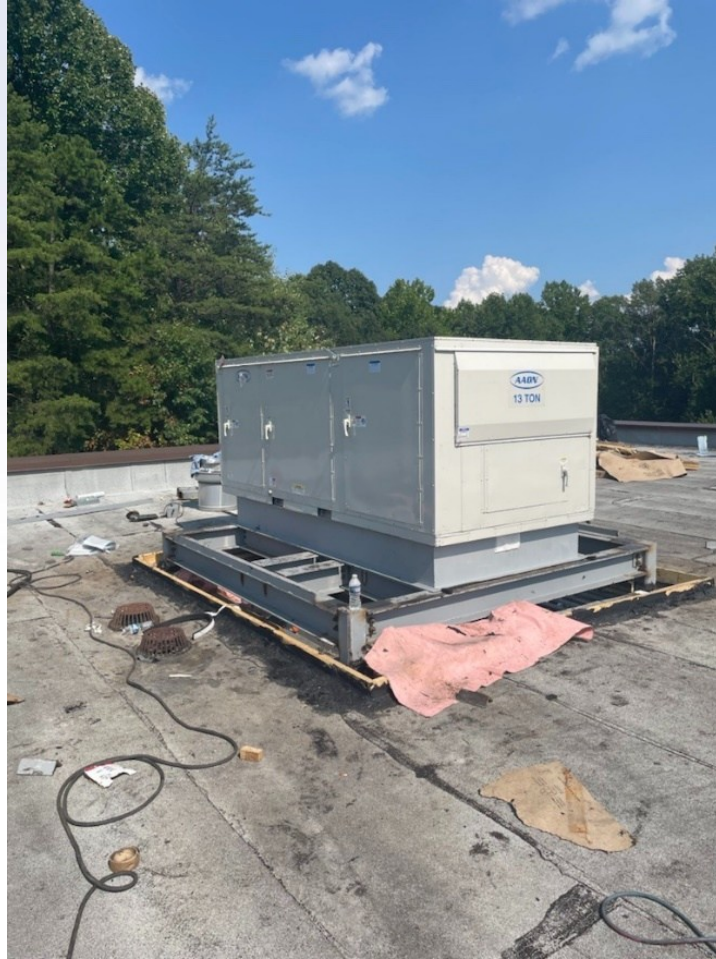
Heavy Infrastructure Renovation
